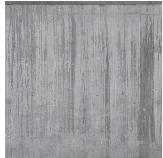
Concrete wall photograph
